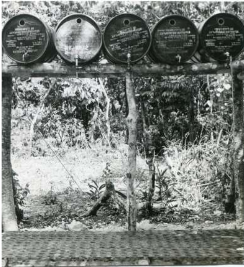
Photograph of a makeshift island shower system, using empty aviation gasoline barrels to hold clean water for showers by American personnel with the 5th Bomb Group, U.S. Army Air Force (from Ferd L. Davis Collection, Military Collection, State Archives).
